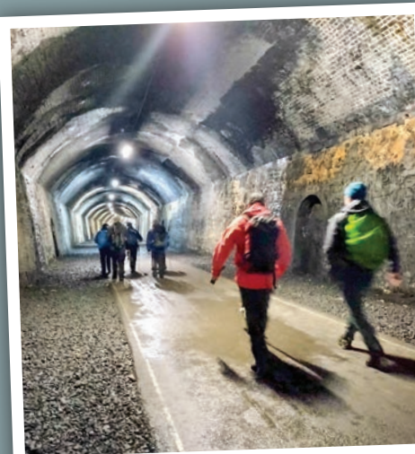
Inside Chee Tor Tunnel – Photograph by Sue Nelson
